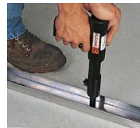
Track to floor
