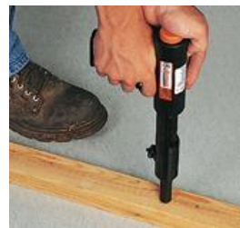
2"x4" to concrete slab
