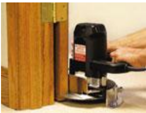
Undercuts Hanging Doors
